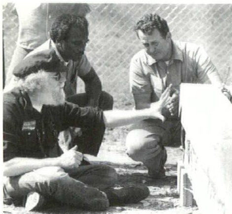
Darrell Henning (left), director of the Norwegian American Museum, Decorah, instructs inmates at Iowa State Penitentiary on the notching of timbers to form half dove tail end joints for the construction of a replica blockhouse of Old Fort Madison.
