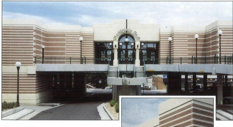
This is precast concrete today! Architectural precast concrete wall panels with a simulated brick pattern.
