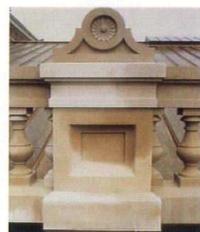
Replacement limestone re-creates the original detail lost to deterioration of sandstone and obliteration by cement-based coatings.
