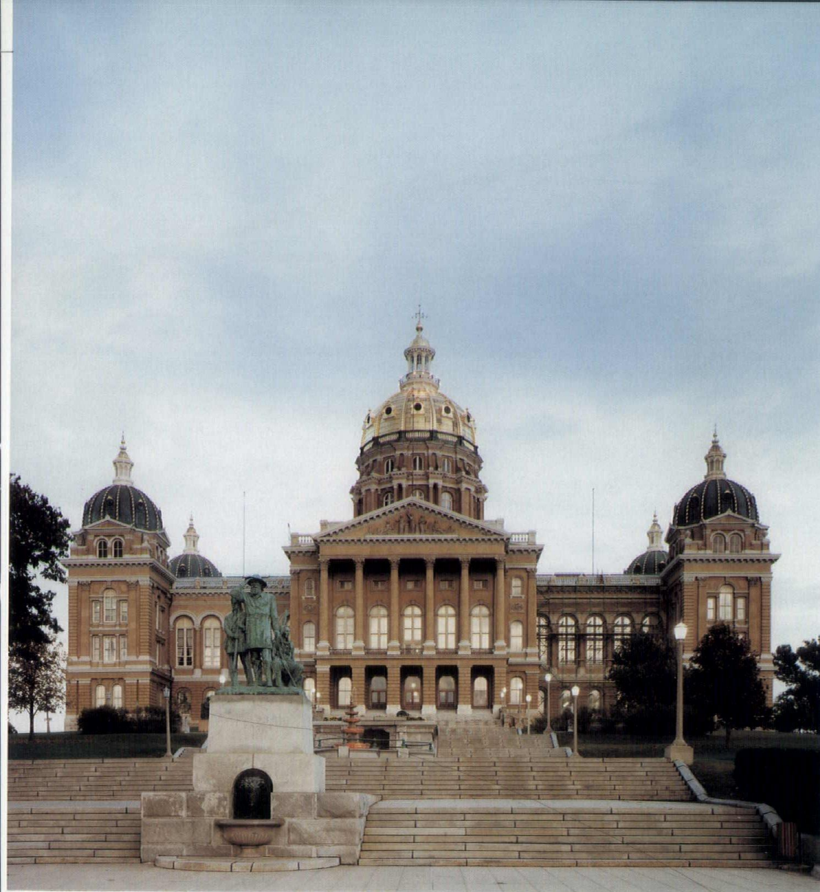
Replacement limestone re-creates the original detail lost to deterioration of sandstone and obliteration by cement-based coatings.
