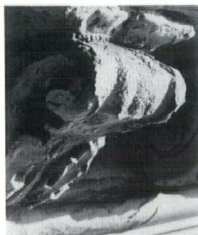
New hand-carved limestone accurately replicates intricate detail. Fortunately a few good examples of these bracket stones still existed for use as models.
