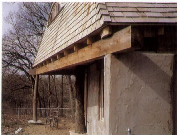
An undressed hickory trunk forms the central structure for the shed's roof.
