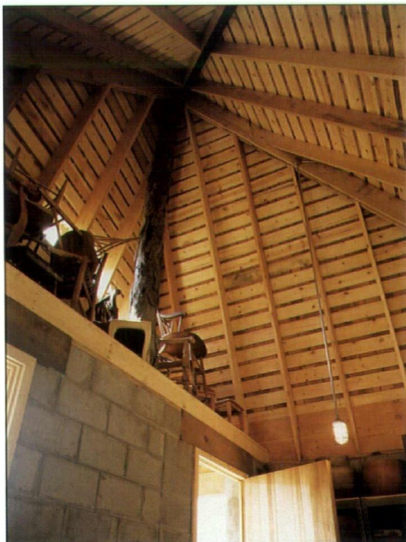
(Right) An undressed hickory trunk forms the central structure for the shed's roof.
