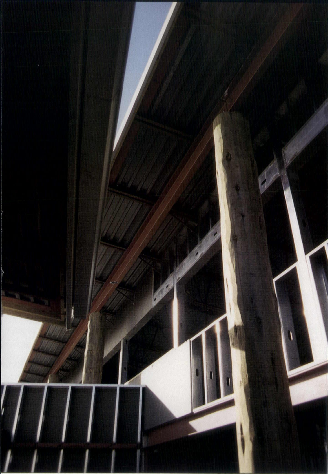
Left and Above: Construction details. Large, rough tree poles, detailed like power poles, form part of the building structure.
