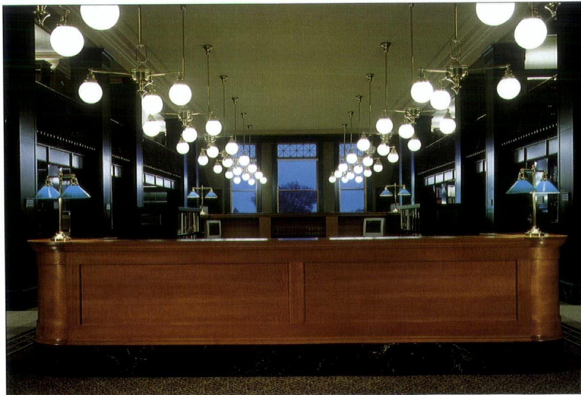
Right: First floor library front desk. Desk reconstructed and lighting manufactured to match original. Mezzanine addition across windows removed.
