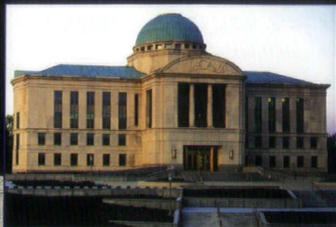
Prairie Foam insulated the 45-ton dome on the new Iowa Judicial Branch Building
