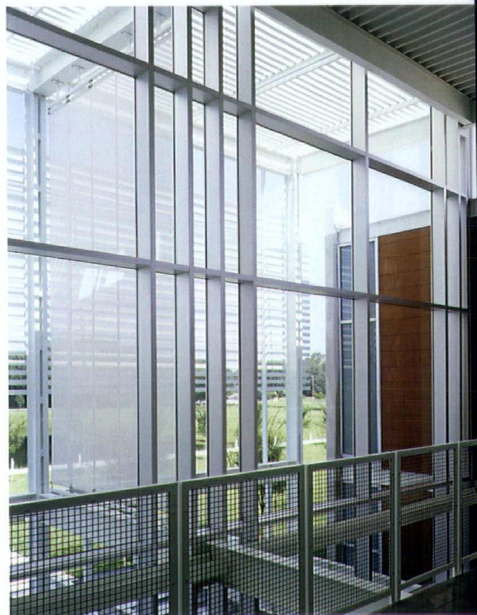
Above: View of the Palmer College's layered lobby cladding. While the inner glass is a conventional curtain wall, the outrigger steel structure and aluminum louvers refer to the environmental traditions of the Sarasota School.
