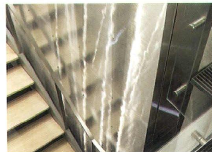
Above: Inside the central conference room, polycarbonate panels provide privacy but also allow the transfer of natural light.
