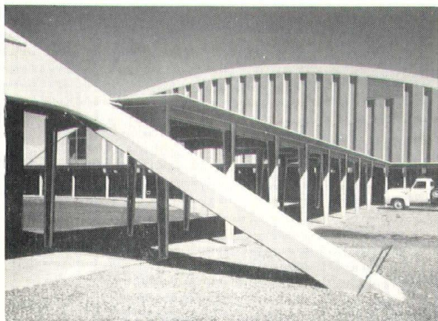
The roof of the multi-purpose building, above, consists of seven 60-ft.-long barrels, each with a 32-ft. chord and 23-ft. radius. Photo below shows the type of covered walks (pre-cast concrete bents) used on the campus. The architect was Maloney & Whitney, Yakima, Wash. The structural engineer was Worthington & Skilling, Seattle. The contractor was Wall, Bartram & Sanford, Wood Village, Troutdale, Oregon.
