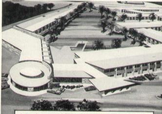
Architect's concept of O'Hare Inn, proposed 535-unit motel now under construction near Chicago's O'Hare International Airport. This handsome structure will utilize Zonolite water-repellent Masonry Fill in block exterior walls, also in cavity walls between rooms. Arch.: Arthur Swanson. Gen. Contr.: John Theodosakis.
