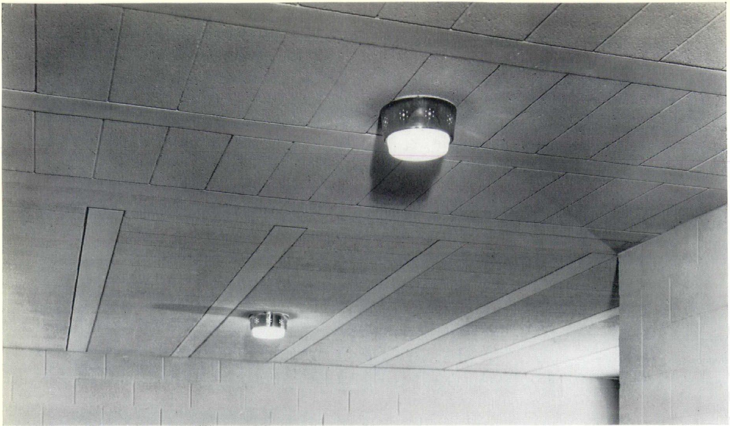
In the Immanuel Methodist Church, Indianapolis, this flush TEE-JOIST ceiling shows how effectively joist can be used perpendicular to each other.
