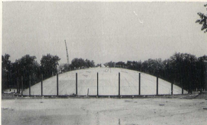
With all concrete in place, the entire dome assembly was allowed to cure and then the five step roofing process began. When lifted into final position 24 feet above ground (at the base of the compression ring), the dome was fully roofed and insulated.
