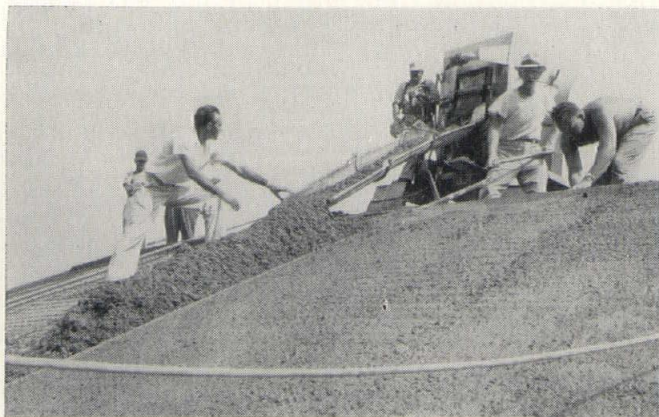
Workmen pour the concrete into one of the sixteen-foot long form sections. 900 Cubic yards of concrete are contained in the dome structure, and the entire dome (including reinforcing steel and compression ring and cords) weighs more than three million pounds.
