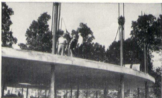
Classrooms coming up! Observing one of the 23 jacks used to lift the roof slab are Gregory Lauer, builder; James McCarron, architect; Dorsey Moss, engineer.
