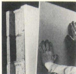
Wall Board Bonding Operation
