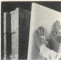
Masonry Wall Bonding Operation
