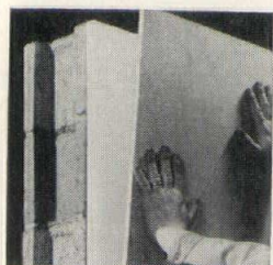
Wall Board Bonding Operation
