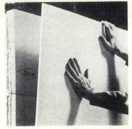
Application of gypsum wallboard over styrofoam SM insulation applied with Dow Mastic No. 11 directly to pre-cast concrete wall panel.
