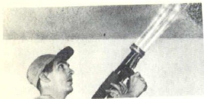
Applied in one operation! Gun sprays dry asbestos fibers which combine in mid-air with water spray.
