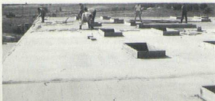
Outside: reinforced, monolithic Zonolite insulating concrete
