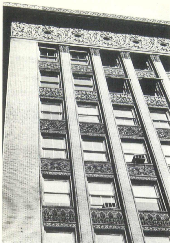
Corner detail of the Wainwright building shows Sullivan's rich ornamentation, executed in dull red terracotta. The attic story has bullseye windows set amid wildly swirling patterns. Note also the fine brickwork.
