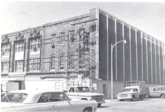
Carthage Texture Vein makes handsome new ground floor facing, while an aluminum solar screen goes over the old walls on the upper floors.
