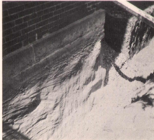
Watkins home showing sub-surface waterproofing applied to the foundation.
