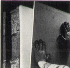
Wall Board Bonding Operation
