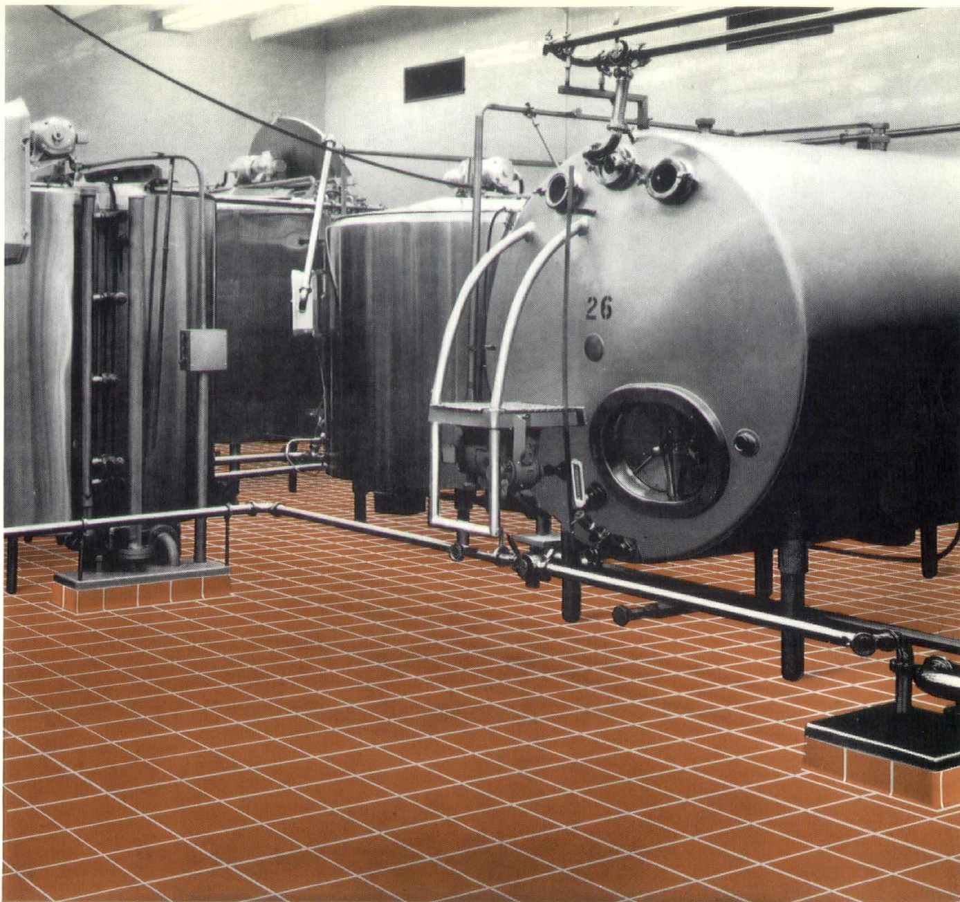
Sealtest Dairy, Louisville, Ky. Floor is Murray quarry tile: 9" x 9" x 3/4" Canyon Red. Architects and Engineers: Johnson & Johnson. Tile Contractor: Rosa Mosaic & Tile. Plate 506.
