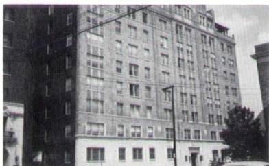
York Towers, Louisville, Ky. Sand Blasted Tuck Pointed & Other Masonry Repairs
