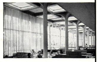
Capturing the spirit of Louisiana traditions in a striking contemporary design, the new Student Union Building expresses the beauty and versatility of modern concrete. Basic concrete structural elements are left exposed to form an intriguing architectural treatment. The reinforced concrete columns, flaring gracefully at the top, provide a single motif for both the interior and exterior of the building.
