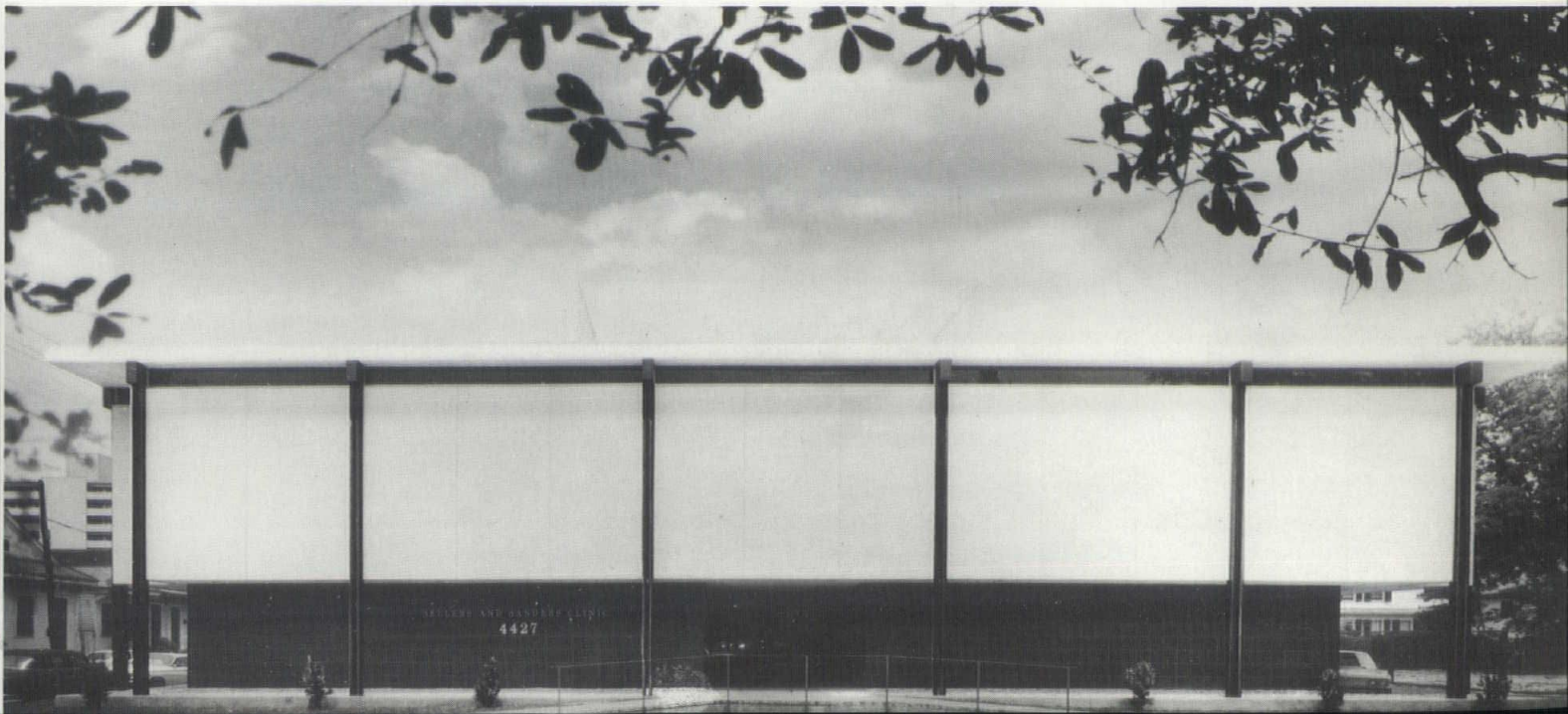
Facade of Tile and Cast Stone Panels, with building-wide overhang protecting entrance.
