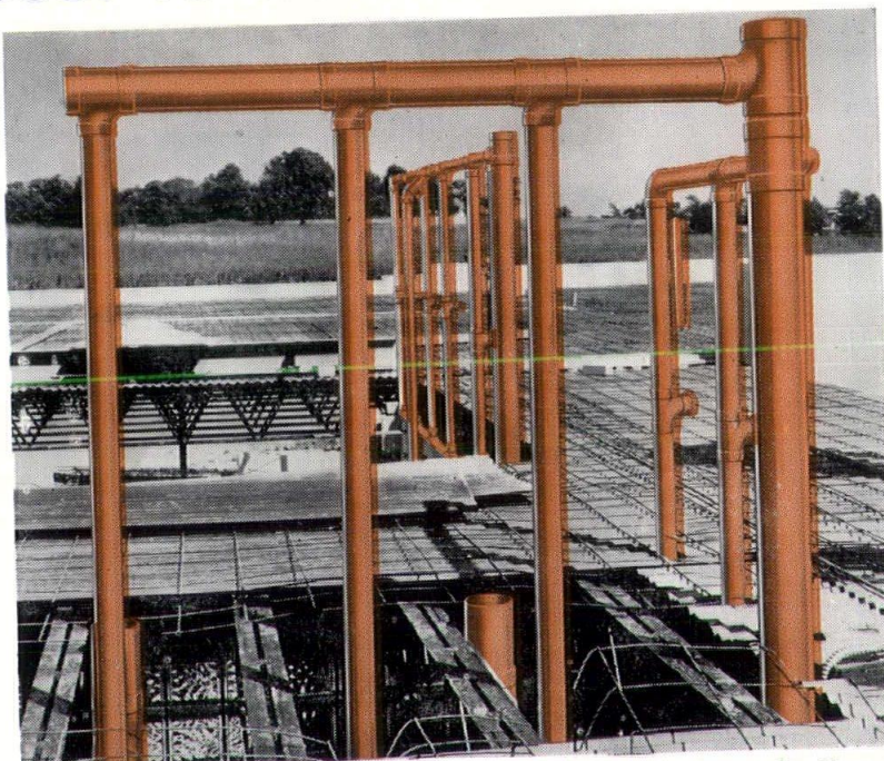
COPPER SANITARY DRAINAGE LINES for second floor lavatories at the Gower School. Light weight of copper tube and ease of making solder joints save many dollars on multiple installations like this. Compact assemblies eliminate wide plumbing walls, give greater usable floor area.
