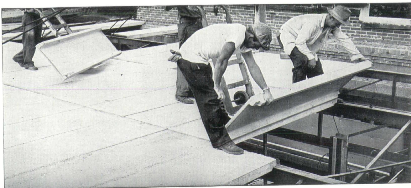
Showing Simplicity of Installation of Truscon Pre-Cast Cement Roof Tile
