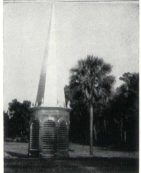
Prefab Steeple and Cupola, First Presbyterian Church, DeLand, Fla. The late George H. Spohn, Architect; Henry P. Whitworth, Supervising Architect, Winter Park, Fla.
