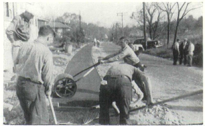
How the cold asphaltic concrete is struck off by means of a screed and then hand rolled.
