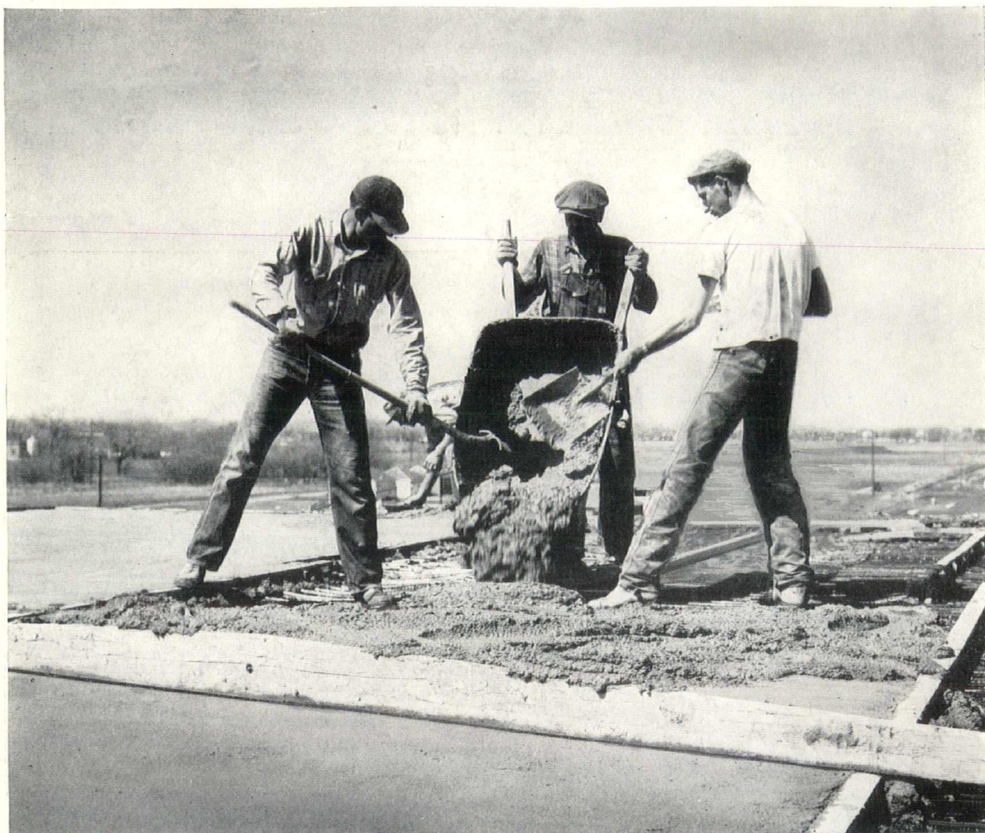
North Platte Junior High School, North Platte, Nebraska, using 5200 bags of Zonolite Insulating Concrete Aggregate. Architect: Davis & Wilson, Lincoln, Nebraska. Contractor: United Builders, Inc., North Platte, Nebraska.
