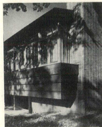
Clear redwood boards create unique inversely stepped glazed balcony.
