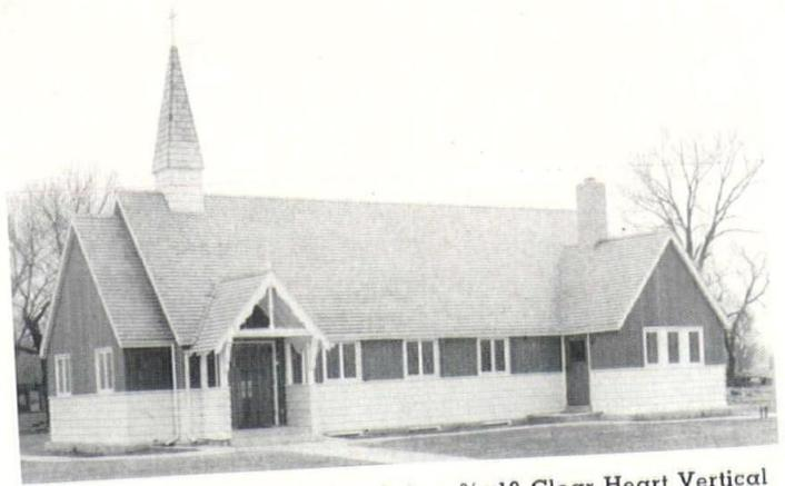
This outstanding small church has  $\frac{3}{4} \times 10$  Clear Heart Vertical Grain PALCO REDWOOD Bevel siding applied on the lower portion and painted white. The same grade of  $1 \times 8$  V-Joint was applied to the upper portion and finished with a natural stain.
