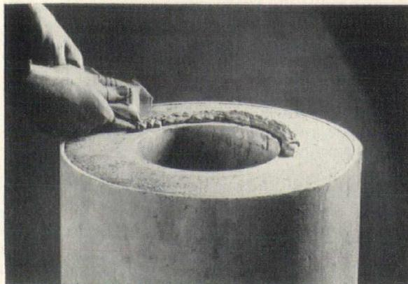
The chimney is listed for all fuels—coal, oil and gas—and all home heating plants and incinerators by UL. The sections are masonry and will withstand temperatures of 2100 degrees F. They provide insulating value equal to a 24-inch solid brick wall or 60 inches of concrete.
