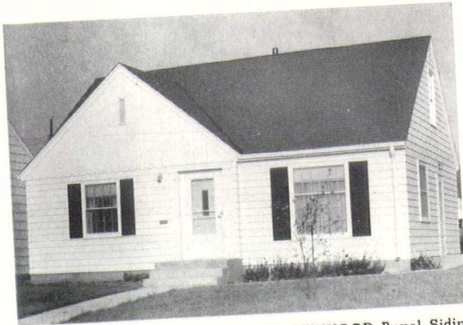
This small home has  $\frac{5}{8} \times 8$ " PALCO REDWOOD Bevel Siding on the walls with a Redwood Board & Batten front Gable. This house was the only one of a 12 house project where the builder used Bevel Siding—and it was the first one sold!
