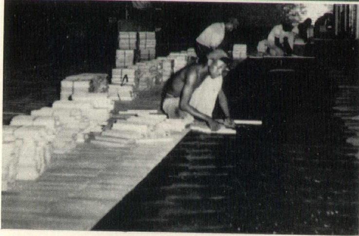
Laid over a concrete slab which was primed and water proofed with Gerrard's #60 asphalt sealer. Set in a full bed of Gerrard's #600 cold mastic.
