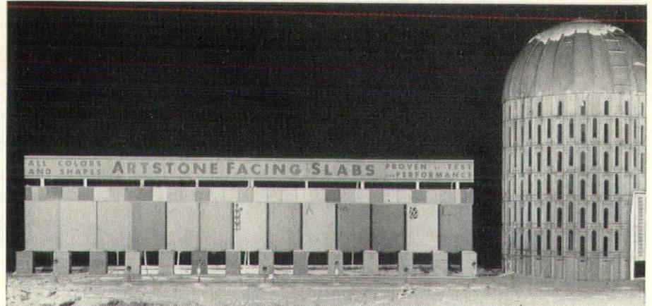
Inspect this display of 61 different Artstone colors exposed in 1938 for weathering observation at roadside in New Ulm's industrial and railroad district.
