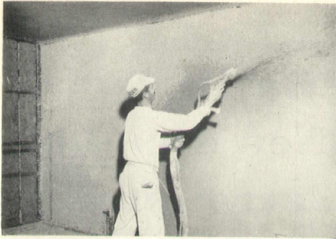
Machine application of vermiculite plaster on gypsum lath for two-inch solid partitions.
