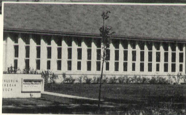
Davidson Architectural Porcelain is used on the Bethlehem Lutheran Church in St. Cloud, Minnesota for the attractive gable at the front and for the "baffle" design between windows on both sides. Smaller picture shows "baffle" treatment from another angle. Architects: Traynor & Hermanson, St. Cloud, Minnesota.
