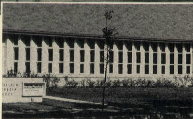
Davidson Architectural Porcelain is used on the Bethlehem Lutheran Church in St. Cloud, Minnesota for the attractive gable at the front and for the "baffle" design between windows on both sides. Smaller picture shows "baffle" treatment from another angle. Architects: Traynor & Hermanson, St. Cloud, Minnesota.
