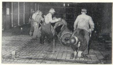
4. Placing concrete is a fast operation. The main positive reinforcement is provided by the deep corrugated steel. T-wires welded across the corrugations furnish the necessary temperature reinforcing and mechanical anchorage between concrete and corrugated steel. Result: A safe, high-strength concrete floor.
