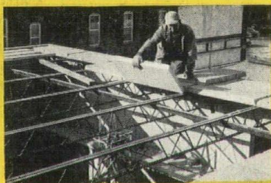
The lightweight (50 lb.) tile, easily handled by one man, is laid directly on the bar joists spaced 36" O.C. forming safe walking surface for workmen.
