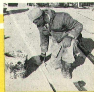
Joints are filled with a quick setting, pre-mixed grout, troweled smooth to provide level surface for roofing. Built-up roof can be applied immediately.
