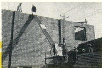
The tile are elevated directly from trailer to roof by means of a powered conveyor as fast as the men can receive them.
