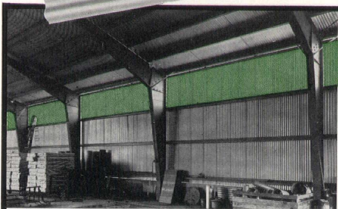
Lasting low cost installation. FILON translucent panels nest with corrugated metal or asbestos. Easily installed, no costly framing.
