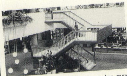
This modern cantilever stairway makes maximum use of precious space and provides an inviting, balcony-like entrance to the store below.
