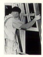
the removal or replacement of sash, weatherstrip and balance at any time during home construction, the company has reported.
