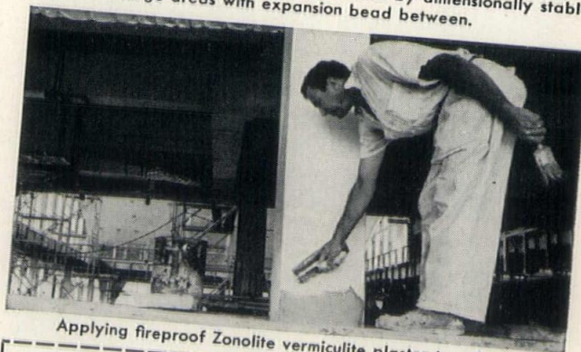
This 204- by 108-ft. clear span parabola was fireproofed with Zonolite vermiculite Plaster Aggregate and sound conditioned with Zonolite vermiculite Acoustical Plastic. Zonolite provided the desired light reflection and expansion was handled by dimensionally stable Zonolite in large areas with expansion bead between.
