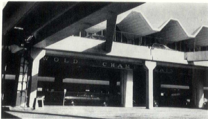
The backbone of the ramp consists of these double-T, beam and column framing materials.
