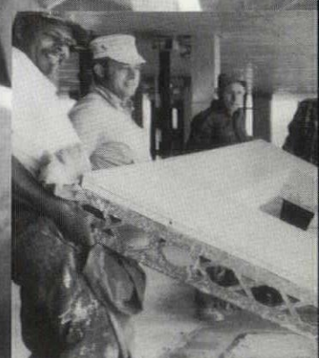
Panel is tilted into place.
