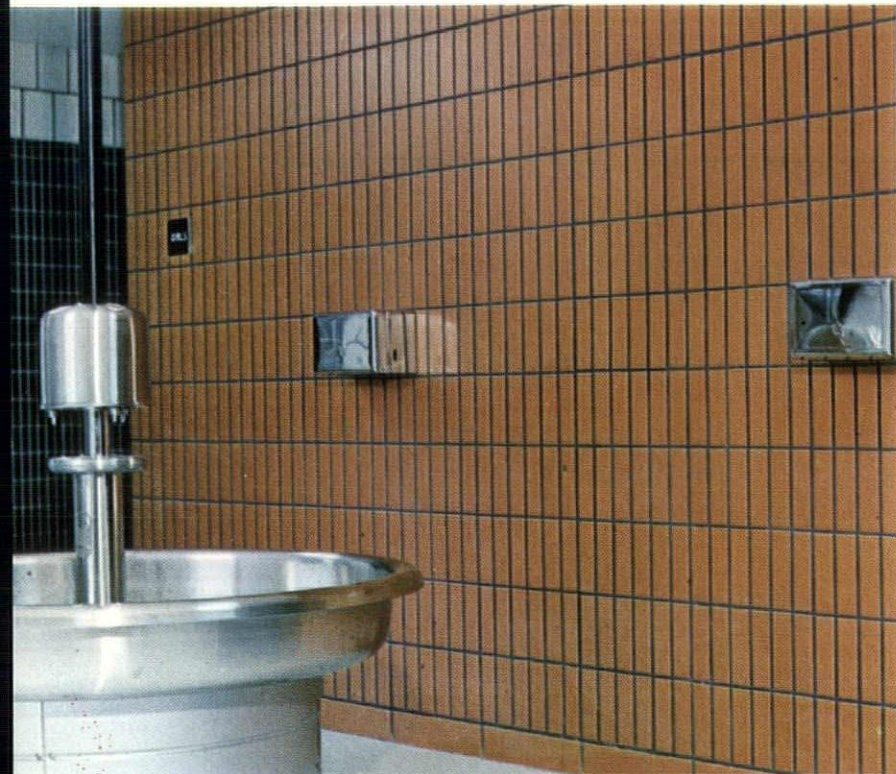
This wall was laid with 8x16 block!
