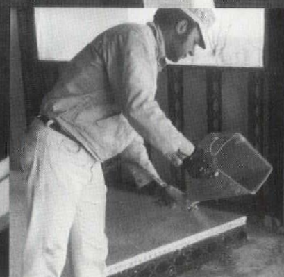
Cement plaster applied. Finish coat is sprayed on.
