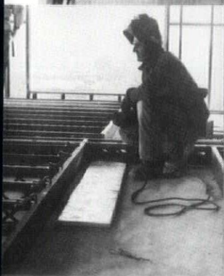
Welder welds studs together.
