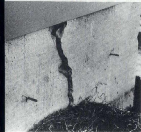
Foundation wall crack.
