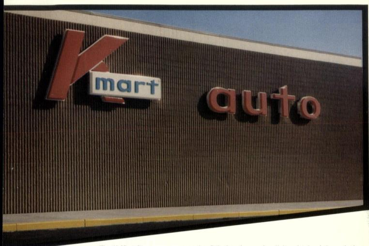
The K-Mart Stores are an example of the handsome simplicity obtained through the of ANCHOR AUTO-CLAVED concrete block. The block used on the K-Mart Stores are an integrally colored reak-off" block providing a unique appearance and low maintenance costs.
