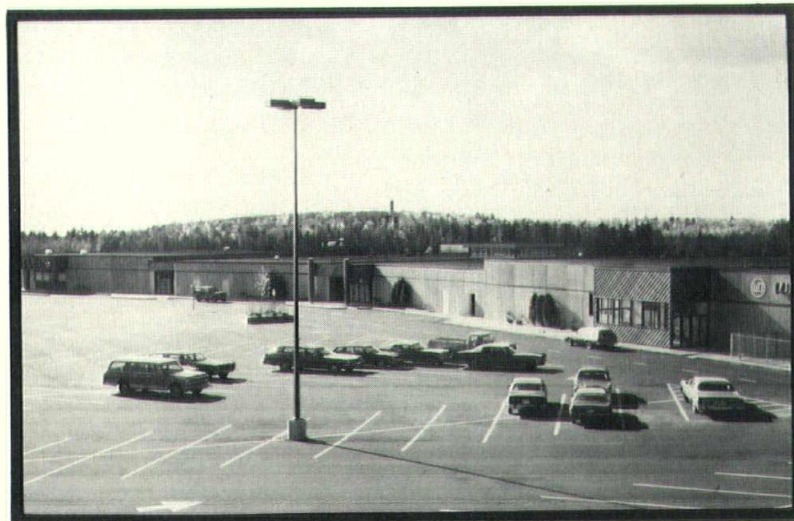
Lumberjack Mall, Cloquet, Minnesota. Designing architect: Roberts Architects, Chaska, MN. Contractor: Ray Riihilaoma Inc., Cloquet, MN. Fabcon's insulated sandwich panels were selected to stand up to northern Minnesota winters.
