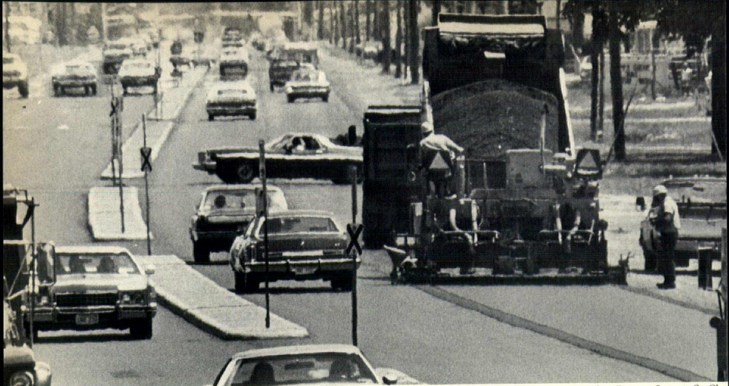
MnDOT 2361 being applied as a resurfacing material on Division Street in St. Cloud.
