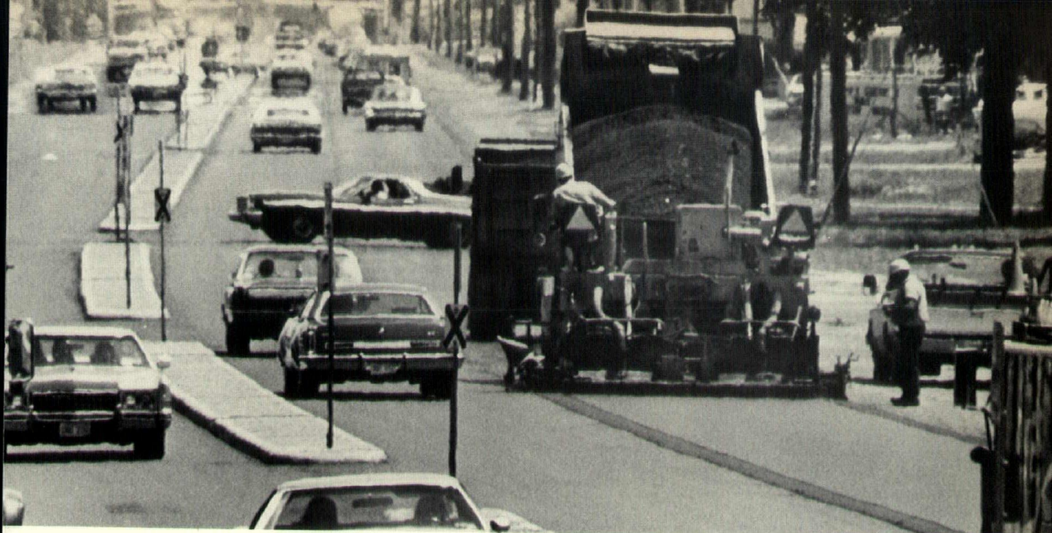
MnDOT 2361 being applied as a resurfacing material on Division Street in St. Cloud.
