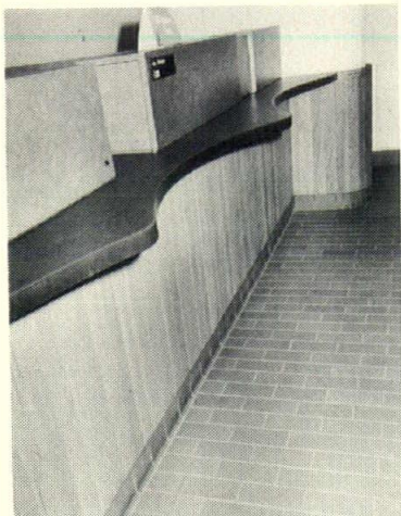
Quarry Tile flooring and Black Slate check desk and ledges. All furnished and installed by
