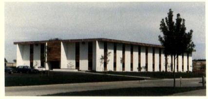
St. Anthony Place Office Building In three short weeks, during the cold of January, Spancrete Midwest Company erected the exterior load-bearing, Corewall panels; 38,000 square feet of Spancrete floor and roof slabs; stair/elevator panels; beams and columns.
