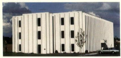
Quebec Plaza The load bearing doubletee wall panel facade combined with interior beams and columns support 14,000 square feet of Spancrete flatslab floor units. The top floor is column-free, because 6,500 square feet of double-tee roof units clear-span the entire building width.
